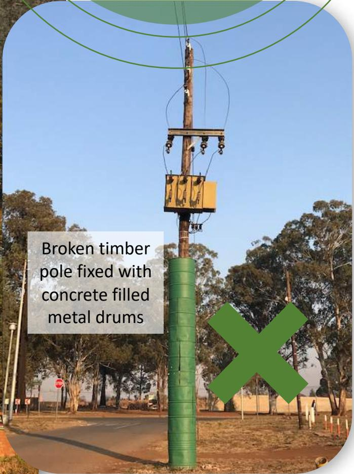
Broken timber pole fixed with concrete filled metal drums
