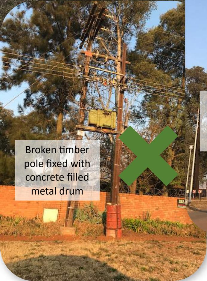
Broken timber pole fixed with concrete filled metal drum
