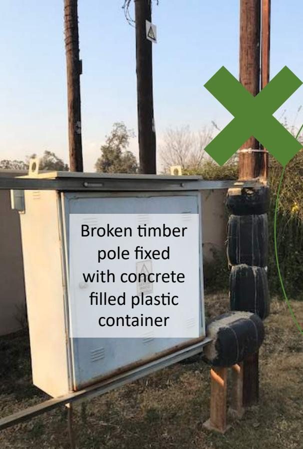
Broken timber pole fixed with concrete filled plastic container
